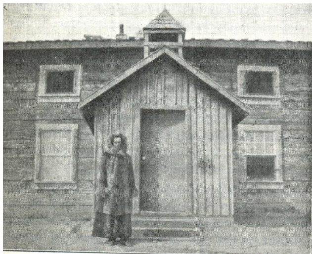
The Bro. Constantin-Marie covered with the "Parkey". T Bro. Constantin's Student Building: On the Ground Floor, Recreation Room, above, the Dormitory
